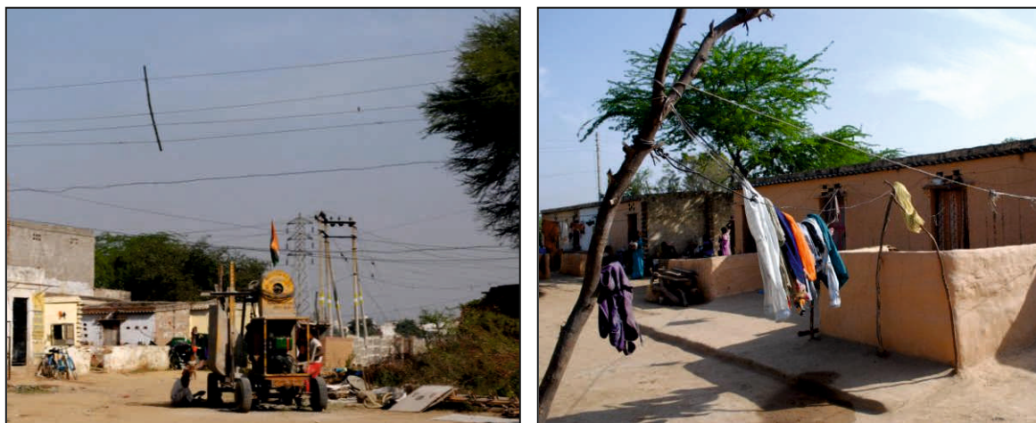
Photograph on the left: shows Perfect Co-existence! - Diesel Genset and Grid Electricity Infrastructure Photograph on the right: shows good (re)use of electric wires to hang and dry clothes in a rural household!
