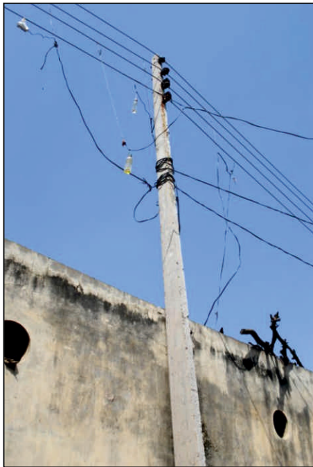
Typical transformer (photo on Right) and Electric poles with wires going everywhere, some for genuine connectivity and some questionable.. (note the water bottles hung on wires in the photograph on the left by people/families opting for electric theft)
