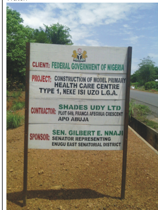
Pic 3: Sign post showing the contract
