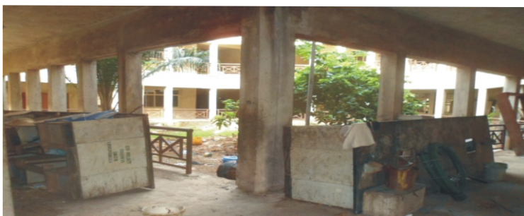
Pic 2: Interior view of the building
