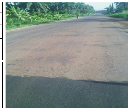
Pic 1: Completed portion of the road
