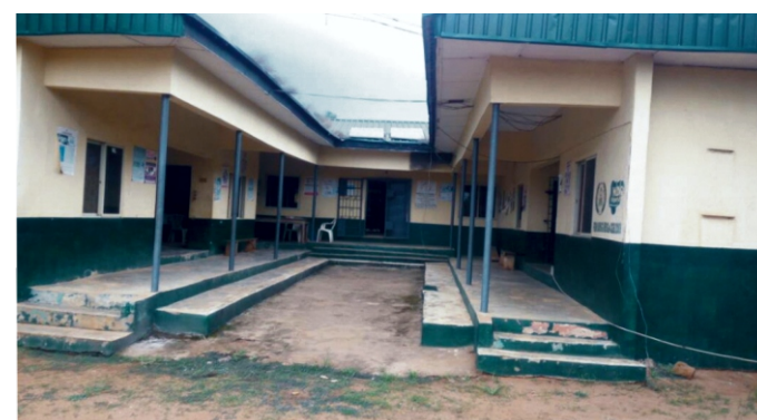
Ukpo Primary Health Care which was constructed before 2017
