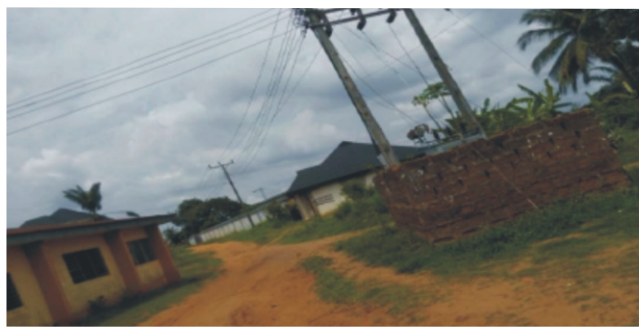
In Amagu Community in Ajalli Community Sec. Sch, Ajalli, No Classroom Block was built at all, No Solar Street Light was installed anywhere. Project Amount is N70M including Umuonyiba, Ufuma in Orumba North FMOWP51908871
