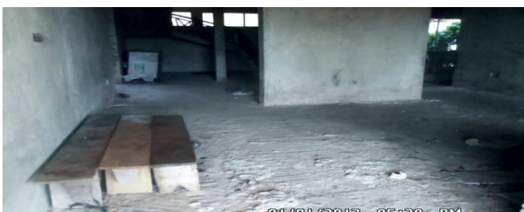
Pic 3: Interior view of the building
