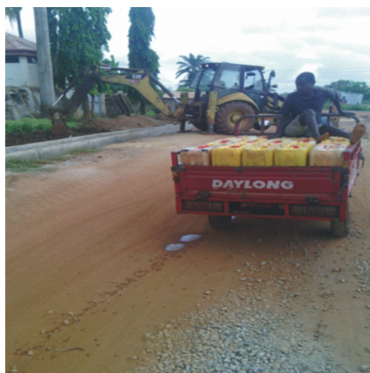
Pic 2: A view of a section of the road under construction
