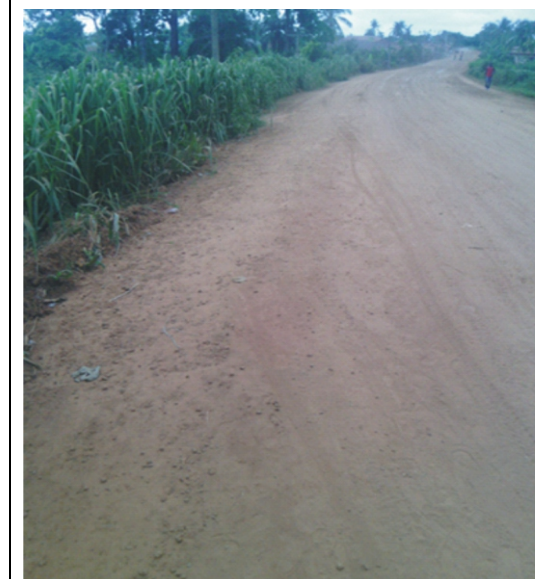
Pic 2: A section of the road under construction
