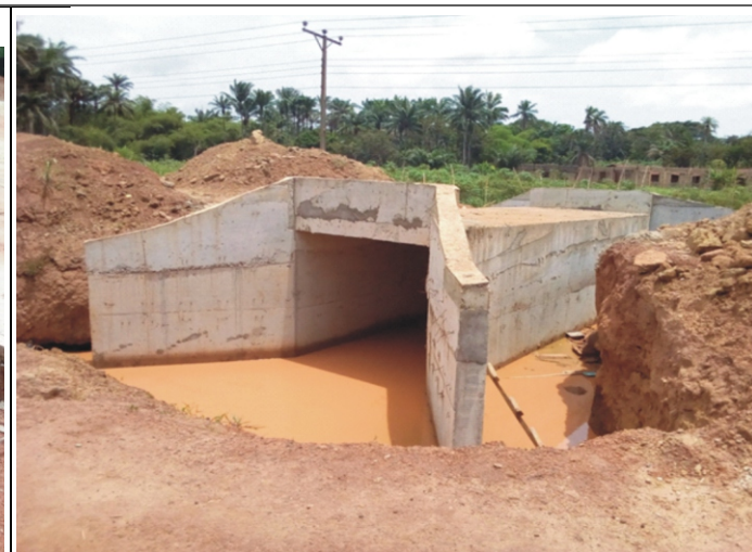
Pic 2: Bridge construction Abaomege-Okposi bridge
