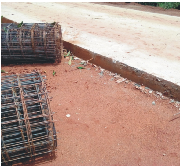
Pic 3: Another view of the road construction
