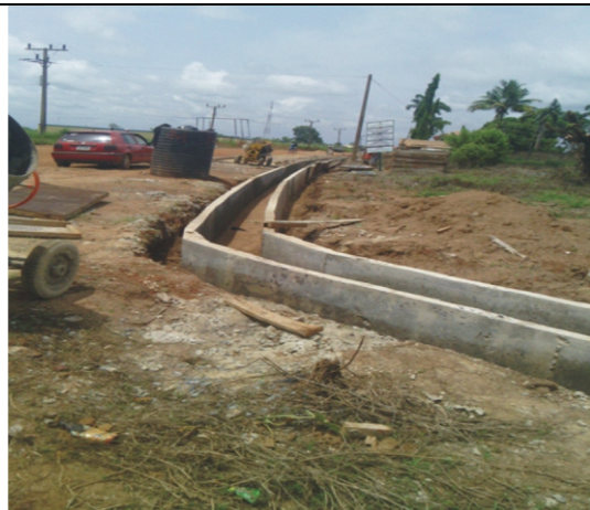
Pic 1: A view of section of the road
