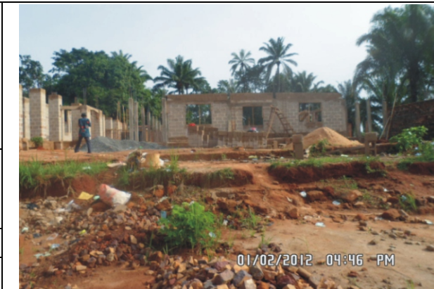
Pic 1: Town hall building construction site at Umuawulu
