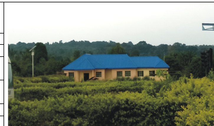
Completed mixed building at ELDI
