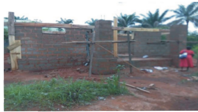
Two Bedroom for PHC Ezinifite (Work in Progress but no fence)
