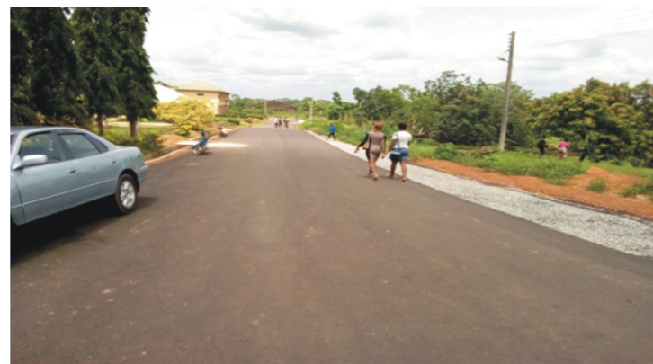
Pic 2: Another view of the road project
