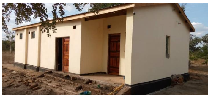
Picture 4: Warehouse at Nkhonde Cooperative
