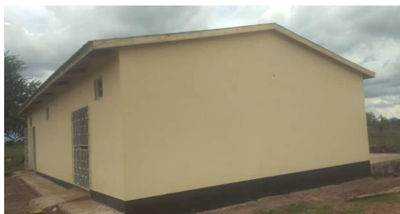
Picture 2: Warehouse at Namibawa in Balaka
